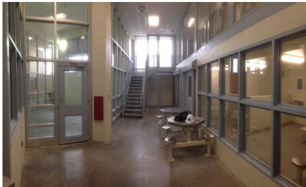
Female Suicide Dorms Douglas County Jail New Health Services Facility (RicciGreene Planning and Architects Design) Photo credit: CGL archives
