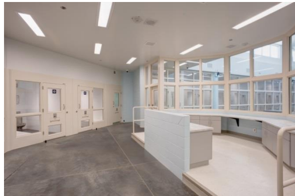
Close Watch Single Observation Cells David L. Moss Justice Center Mental Health Expansion for Tulsa County (Dewberry Architects Design) Photo credit: Jon B. Petersen Photography, Inc
